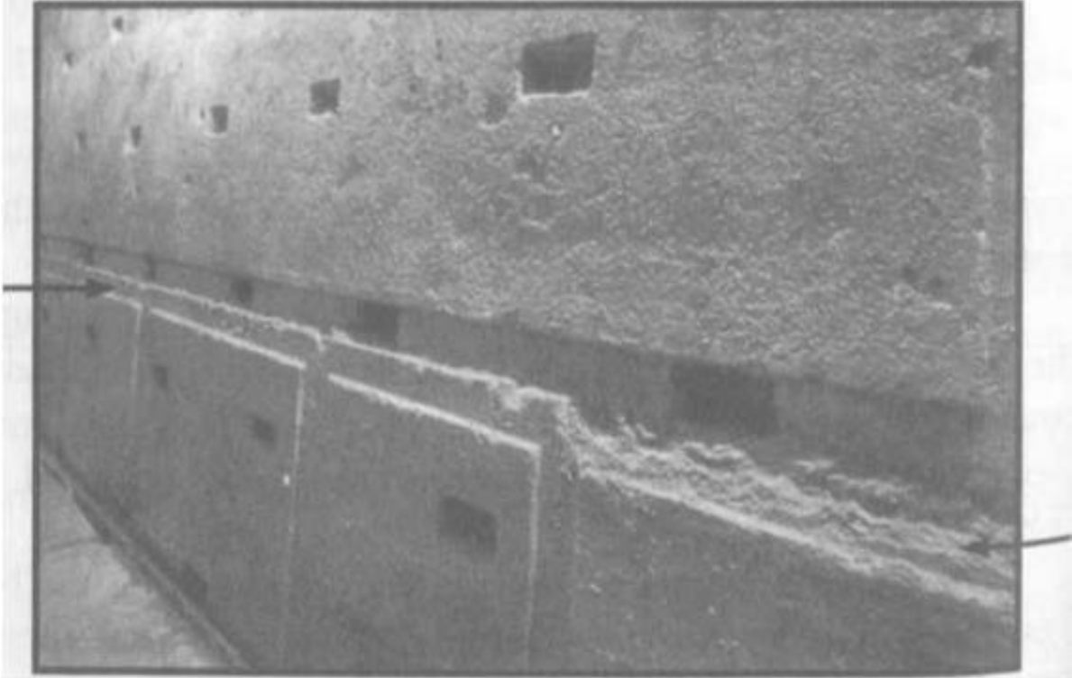
The photo above shows the Herodian stones with the handsbreath border around the edges.
