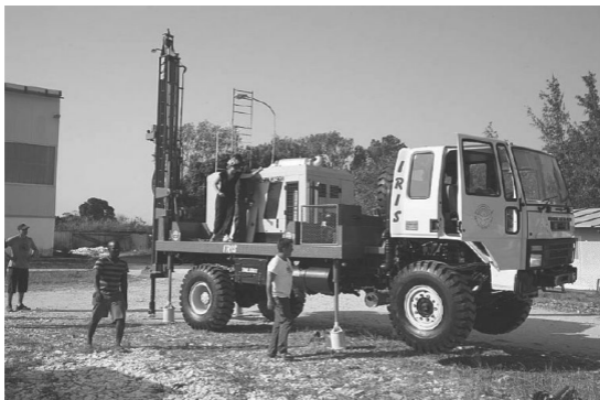
In position for drilling
