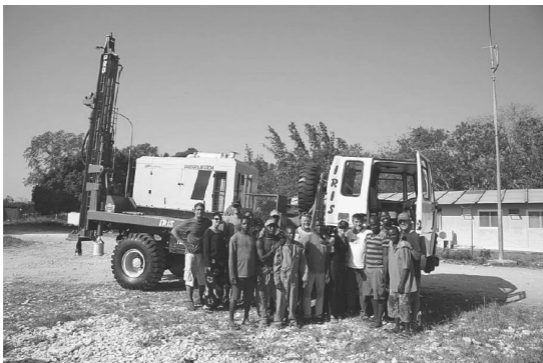
Auxiliary truck with water tank, pump and drill bits
