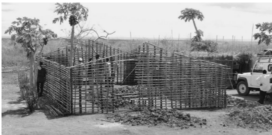
The framework of a new church building coming together
