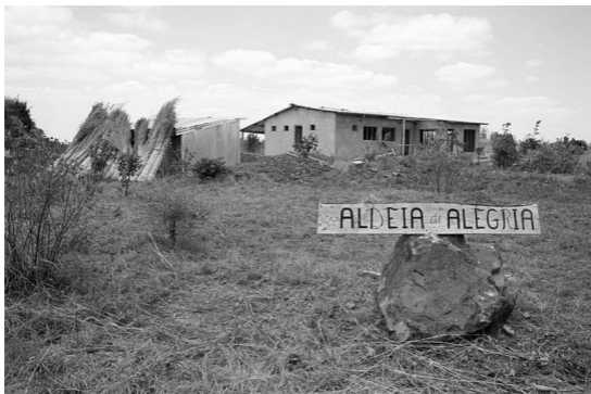
Building a dorm for our new center in Lichinga, Niassa Province
